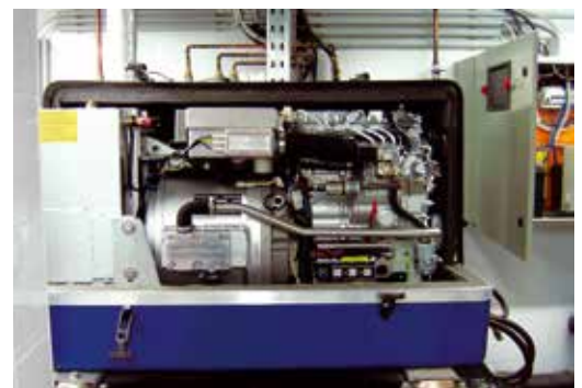
This three-phase Panda is installed in the basement. Main fuses, panel and radiator control are fitted in electrical cabinet. Image: Kratos Kft. Hungary.
